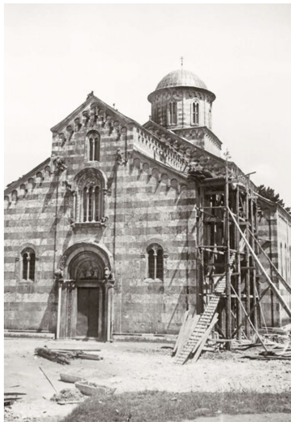
Dečani, scaffold on the south façade of the narthex (Documentation of the Visoki Dečani Monastery, F234)
